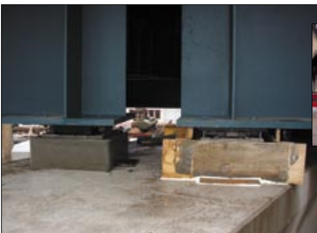
Chemnitz-Einsiedel viaduct, Blankenauer street: repairing bridge bearings
