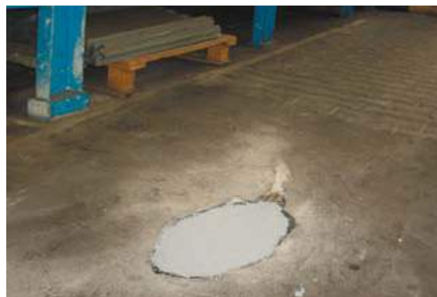
Renovation of flooring in a rolling mill
