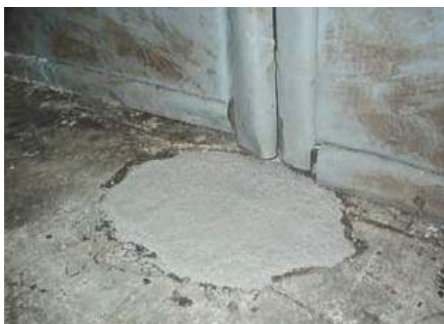
Improvement of the flooring in a cold store in continuous operation with SILIKAL® R 17 (-25 °C) mortar
