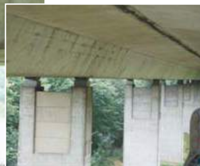
Renovation of the bridge bearings of a motorway bridge
