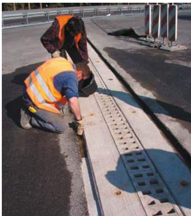
Installation of the lateral drainage channels in a motorway
