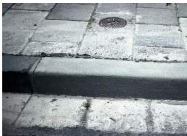
Renovation of kerbstones with SILIKAL® R 17 mortar
