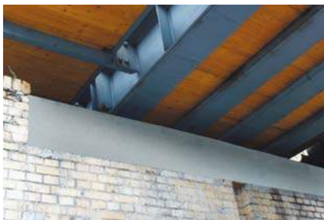
Renovation of the bridge abutment of an urban railway bridge
